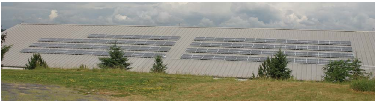
Albany County Hockey Facility Solar Panels (with permission from Albany County)
