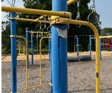
Playground equipment is deteriorating.
