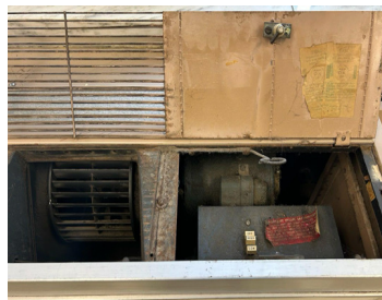
HVAC units are nearly 60 years old and are failing or obsolete.
