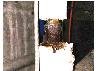
Plumbing infrastructure is aging and deteriorating.
