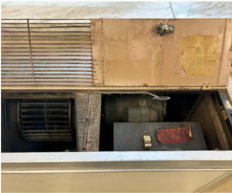
HVAC units are nearly 60 years old and are failing or obsolete.
